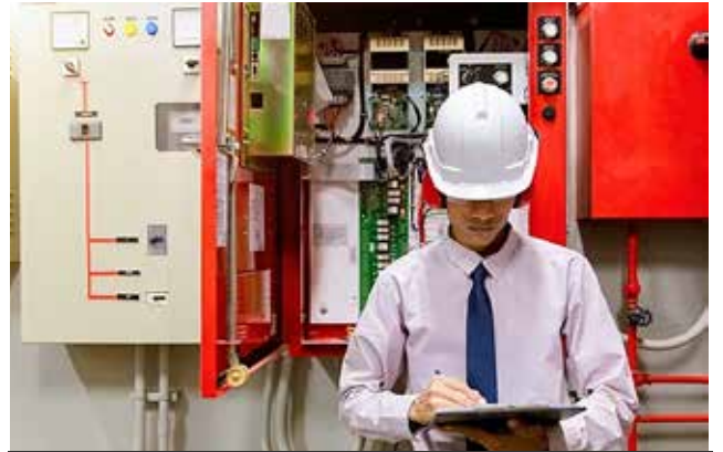
Test Ve Devreye Alma Sistemleri Testing And Commissioning Systems
